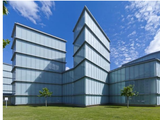
FIGURE 4. SIDE OF THE BUILDING
