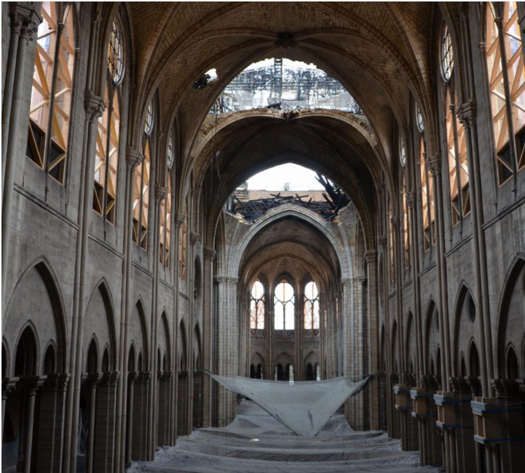
The nave and vaults destroyed in the fire © Maxime L'Héritier - Metal Working Group
