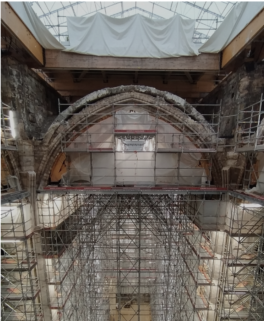
The scaffolding in the nave seen from the crossing © Maxime L'Héritier - Metal Working Group
