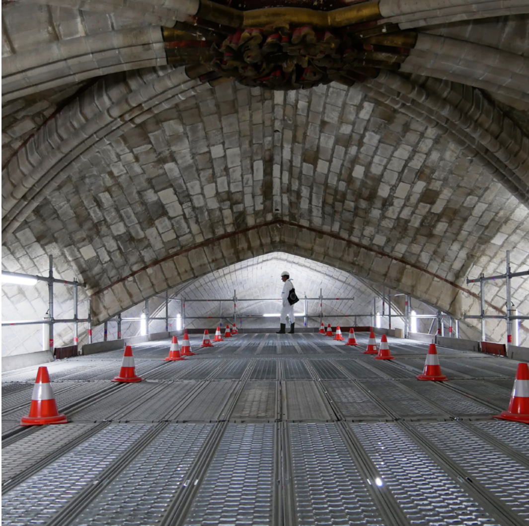
Access to the vaults using scaffolding © Elise Baillieul - Stone Working Group
